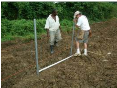
Figure 3 Foundation stake measuring rod
