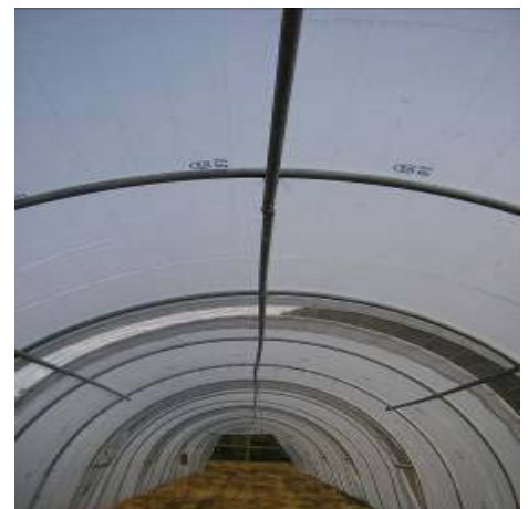
Figure 7 Completed center brace pipe
