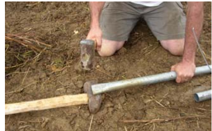
Figure 10 Flattening end of side pipe
