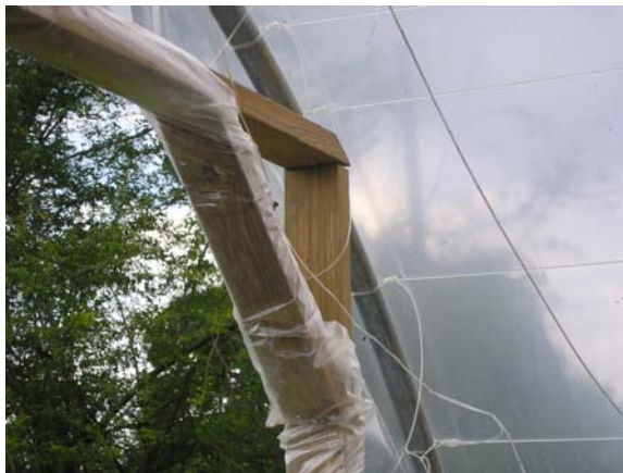
Figure 31 Top, side and angled door brace frame
