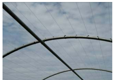
Figure 17 Monofilament line across top of HTH
