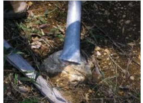
Figure 2 Crimping foundation stake point
