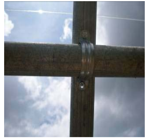
Figure 8 Installed center brace pipe straps with two self-tapping screws
