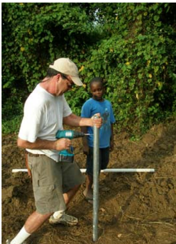
Figure 6 Screwing in self-tapping screw
