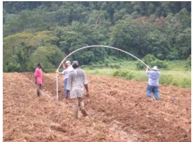
Figure 5 Installing hoop pipes into foundation stakes
