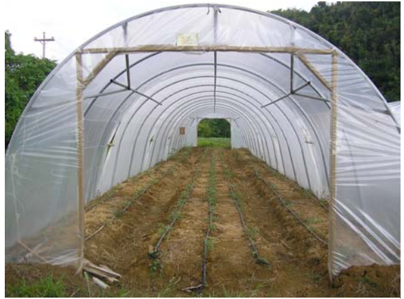
Figure 32 Exterior plastic secured to door frame
