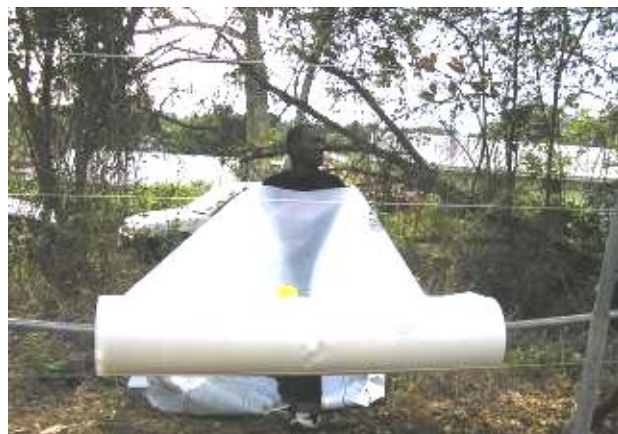
Figure 11 Pipe roller placed on two ladders
