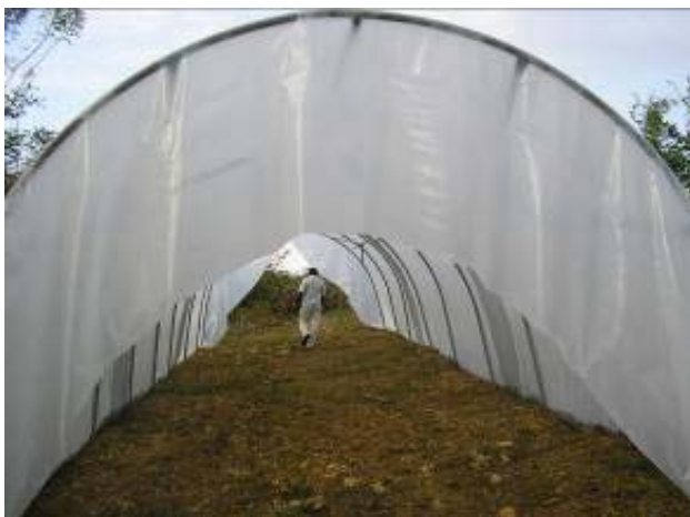
Figure 30 Plastic overlap front & back to attach to frame
