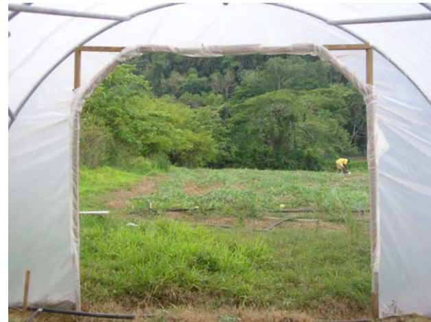
Figure 33 Interior plastic secured to door frame
