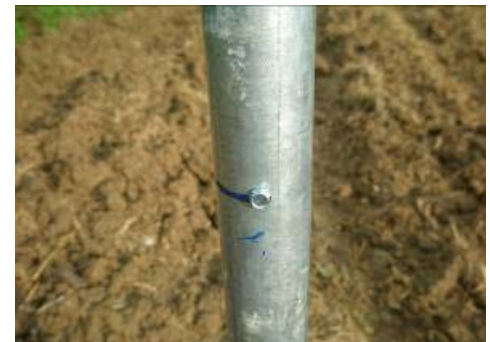
Figure 5 Six inch mark for self-tapping screw
