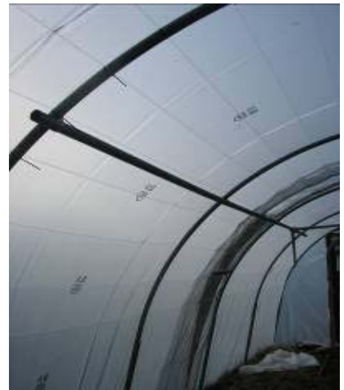
Figure 9 Side pipe brace connected to hoops 2 & 5
