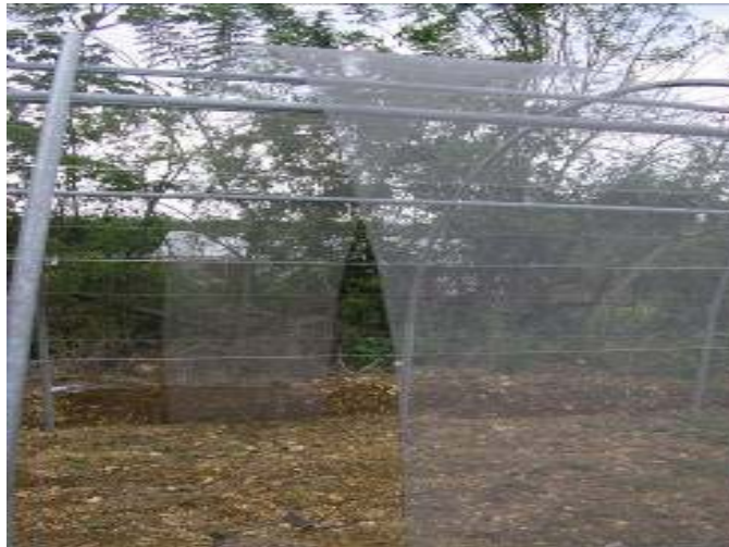
Figure 23: Mesh is installed and buried in the trench
