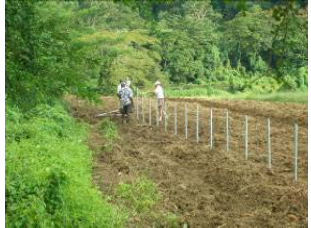
Figure 4 Leveling and marking foundation stakes
