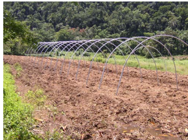
Figure 6 Complete hoops in foundation stakes
