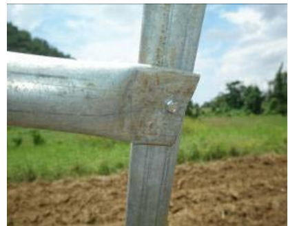
Figure 13 Side brace flattened on end for screw connection
