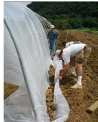
Figure 20 Careful back filling of trench to bury and anchor mesh & plastic cover
