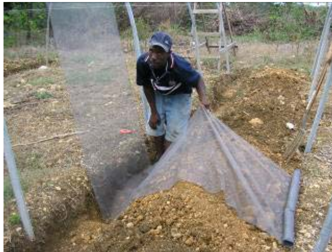
Figure 21: The mesh is stretched tight over the HTH
